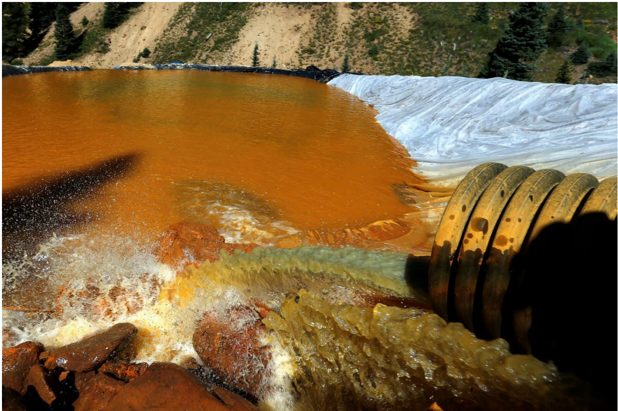
In this Aug. 14, 2015, photo, water flows through a series of sediment retention ponds built to reduce heavy metal and chemical contaminants from the Gold King Mine outside Silverton, Colo.
