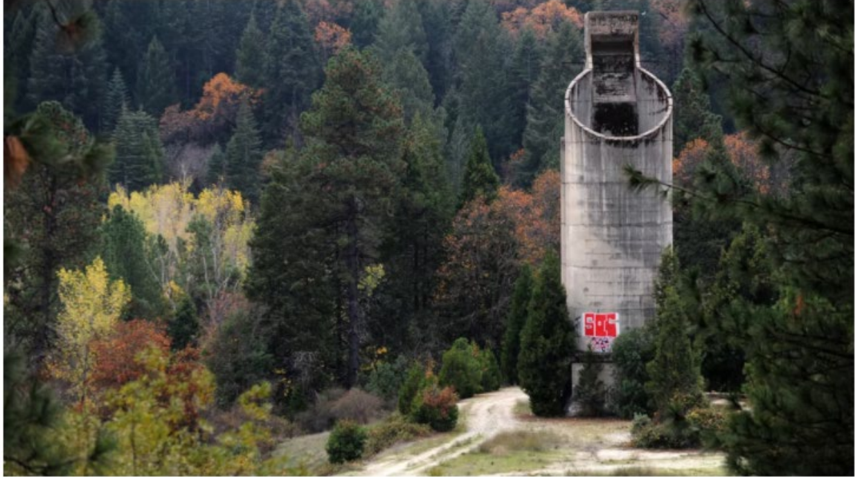
Grass Valley's Idaho-Maryland Mine, abandoned for nearly 70 years, is marked by a weathered concrete silo. (Becki Robins)
