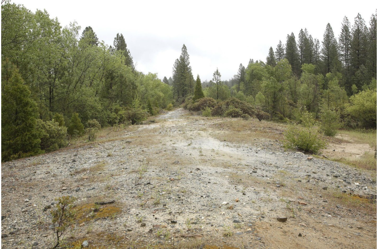
An arsenic-laden tailing berm near the site of the abandoned mine. (Elias Funez / Union)
